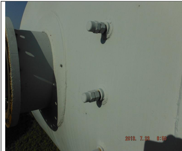
Couplings welded to shell
